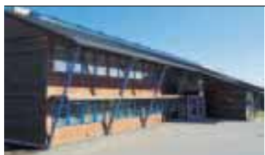
STEMA/PEDAX Headquarters – Denmark
