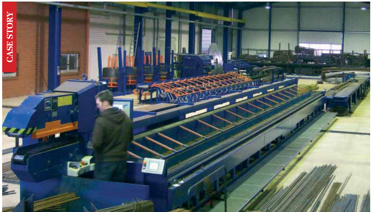
Richters new hall with Metax Geco rebar shearline.
