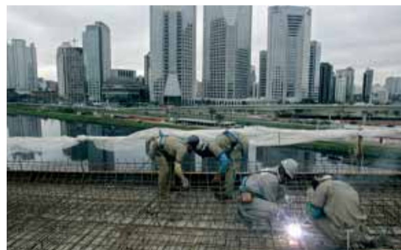
Buildings under construction in São Paulo
